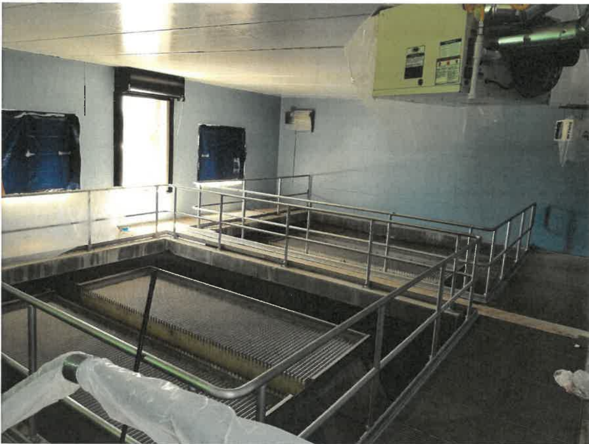
Water Treatment Plant Renovation – Photo by Scott Hoover
